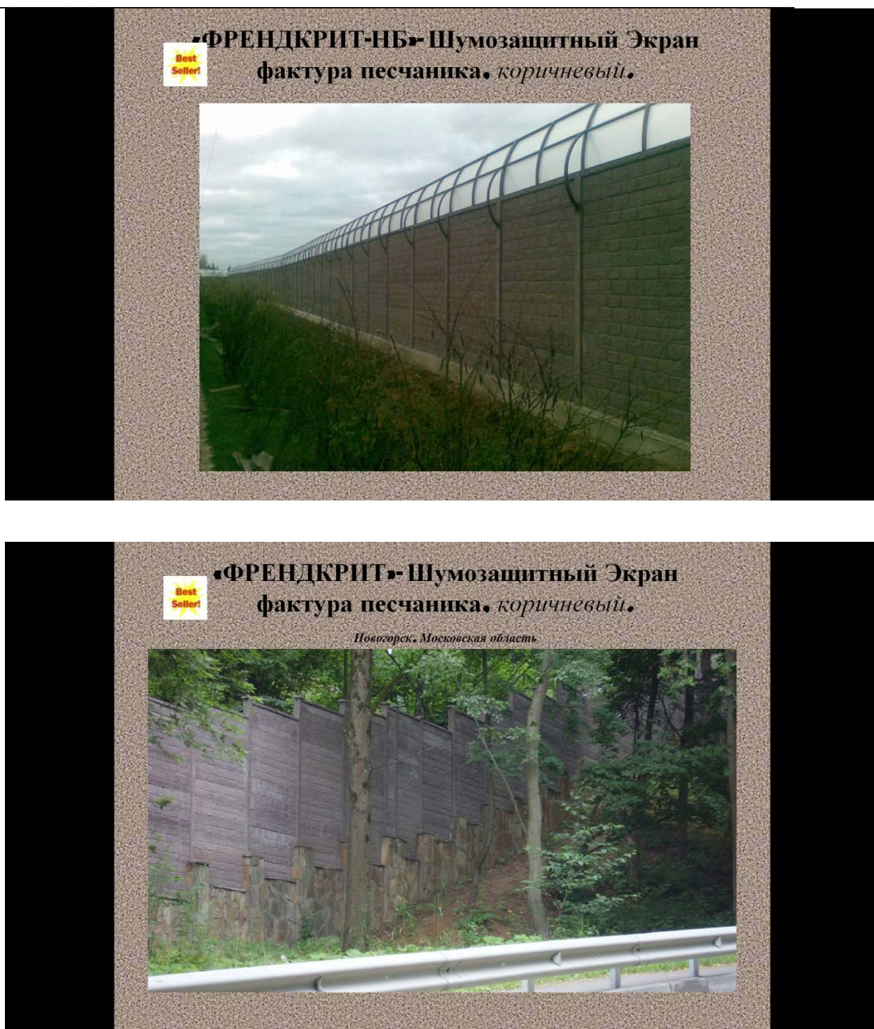
Fig.7.6., 7.7. Noise Barriers Mounted Using Concrete Slabs
