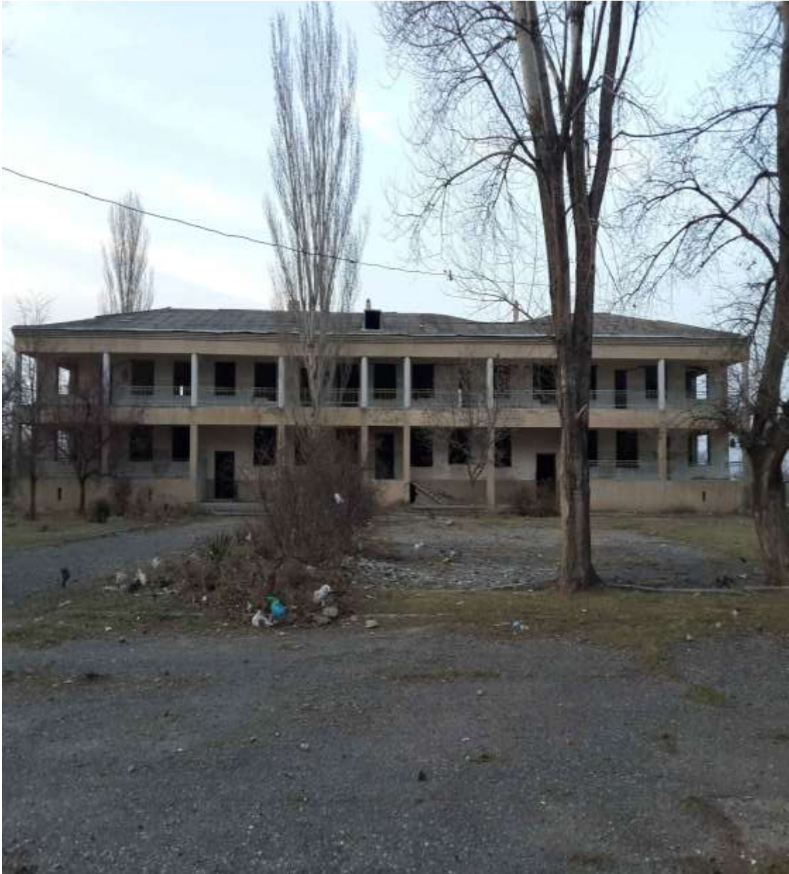
Pictures of the existing building
