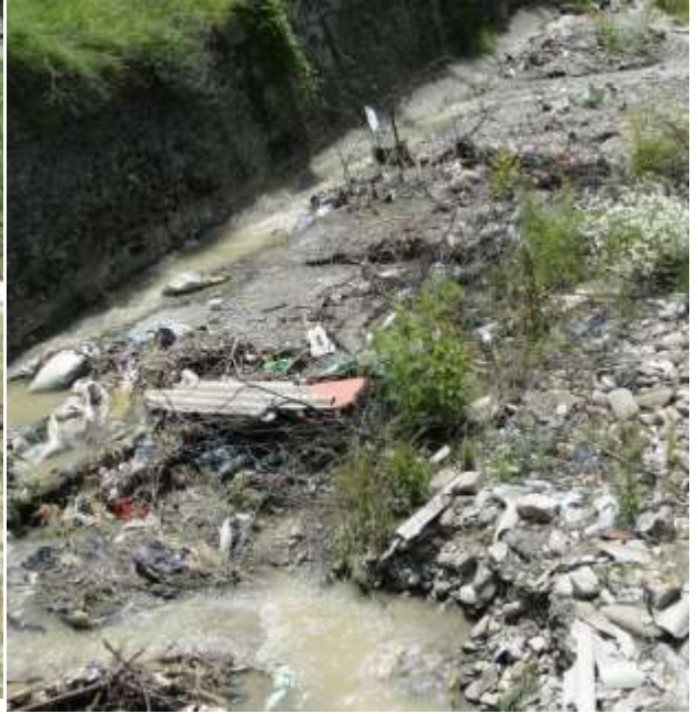
Current condition of "Telavi Khevi" bed
