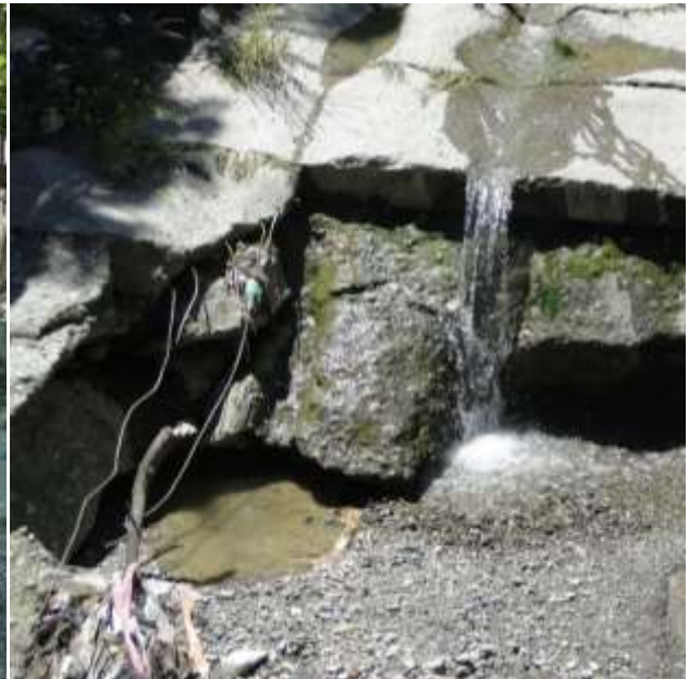
Current condition of "Telavi Khevi" bed
