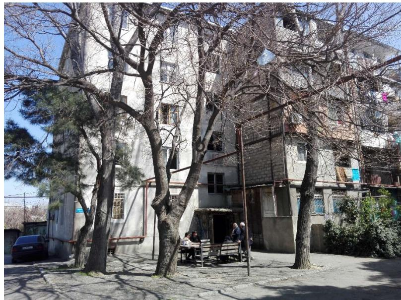
Building 5 is composed by three different blocks, separated by a seismic joint. Each block is disconnected, so three different monitoring were necessary.
