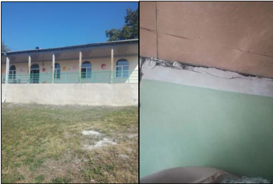
Figure 7 Photos of existing kindergarten building
