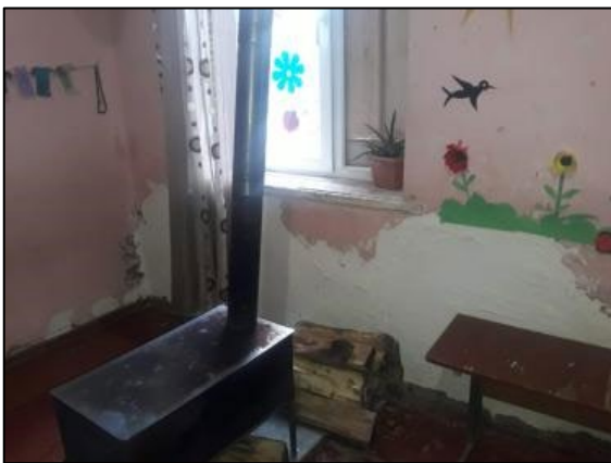
Figure 7. Photos of existing kindergarten building
