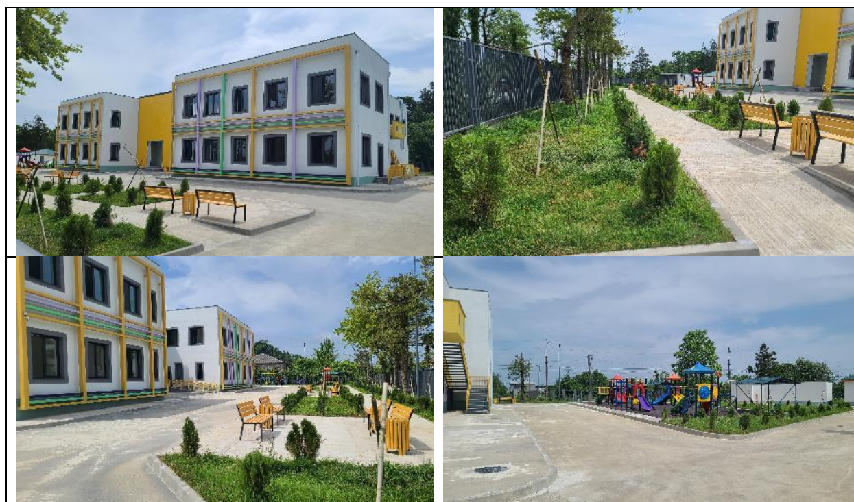
Figure 24 Photo materials reflecting the ongoing civil works
