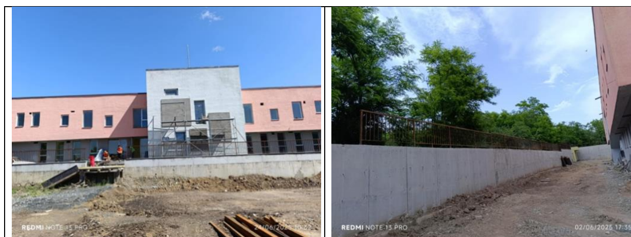
Figure 19 Photo materials reflecting the ongoing civil works
