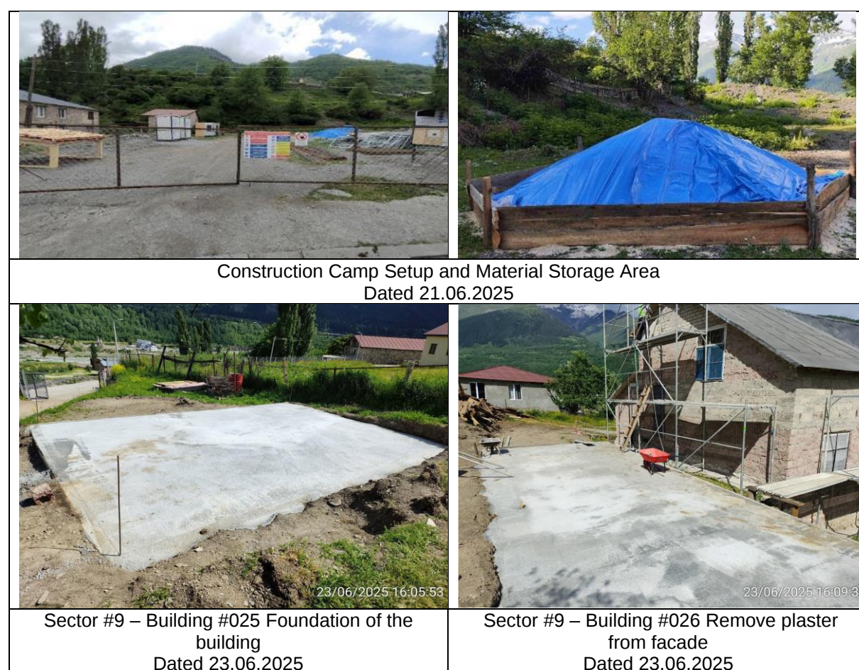
Figure 40 Photo materials reflecting the ongoing civil works
