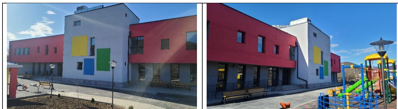
Figure 37 Photo materials reflecting the ongoing civil works
