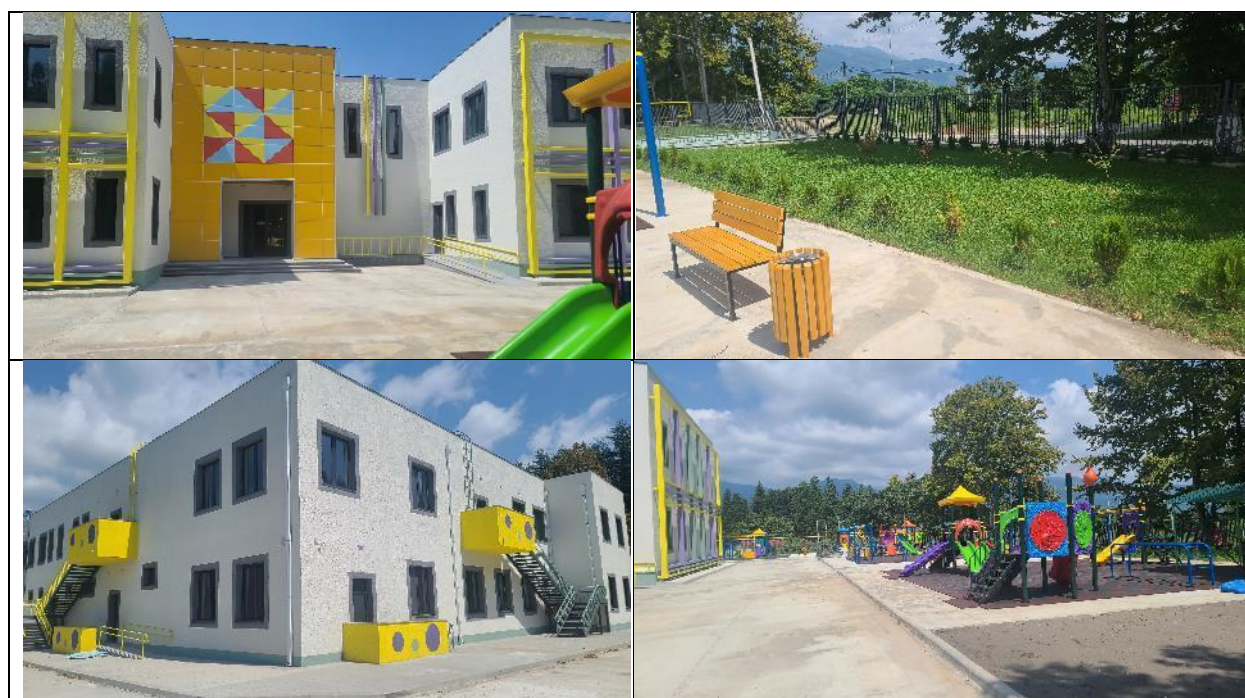
Figure 25 Photo materials reflecting the ongoing civil works
