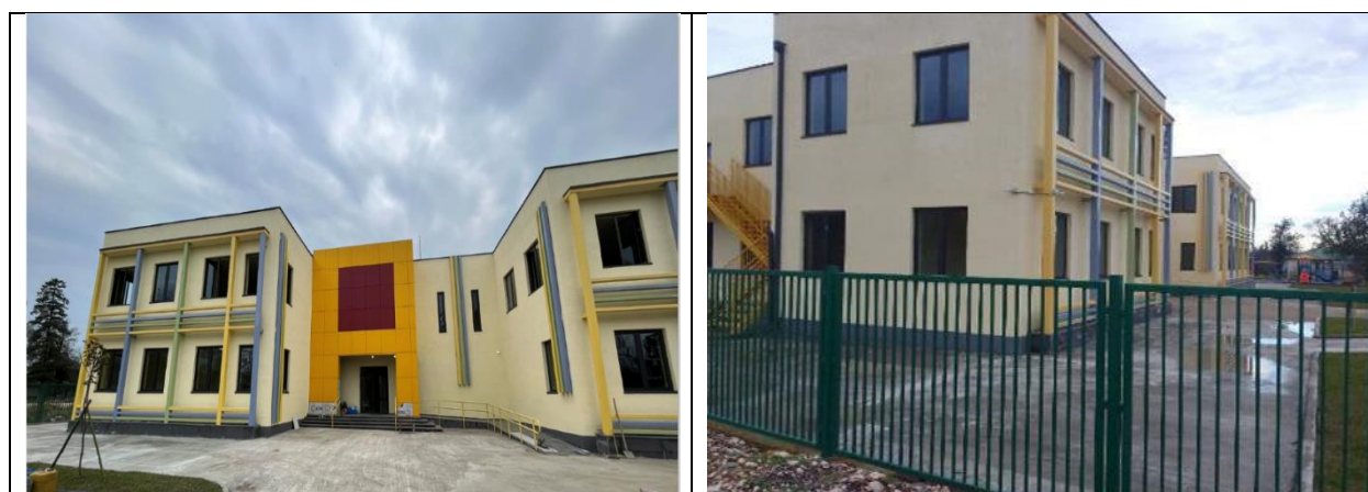
Figure 30 Photo materials reflecting the ongoing civil works
