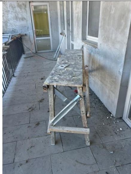
Status: (open, In progress, closed) - Open
