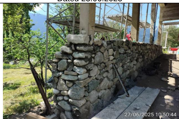
Sector #9 – Building #030 _Arrangement of cement mortar on the Façade Dated 25.06.2025
