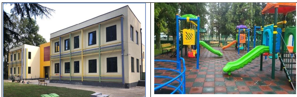
Figure 31 Photo materials reflecting the ongoing civil works
