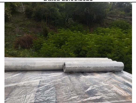
Asbestos-containing pipes securely double-wrapped in plastic sheeting and temporarily stored on a waterproof protective barrier prior to transport to a licensed hazardous waste facility. Dated 27.06.2025
