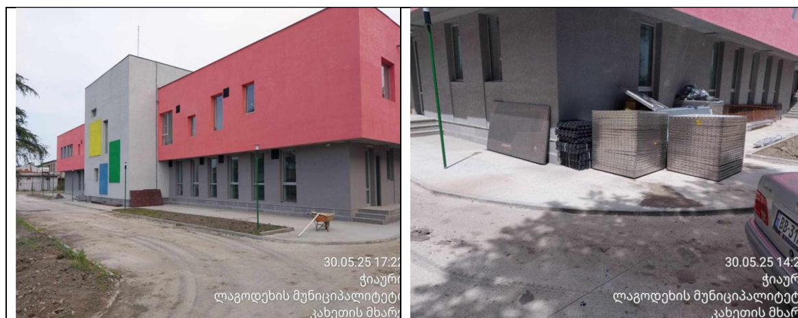
Figure 20 Photo materials reflecting the ongoing civil works
