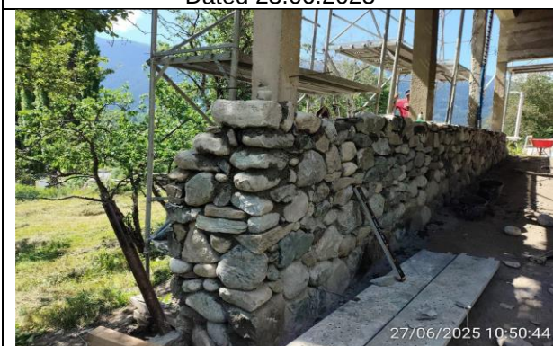
Sector #9 – Building #029 _Finishing of the wall in the front façade with stone Dated 27.06.2025
