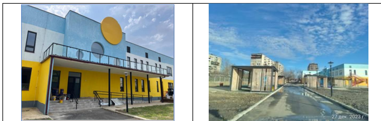
Figure 22 Photo materials reflecting the ongoing civil works
