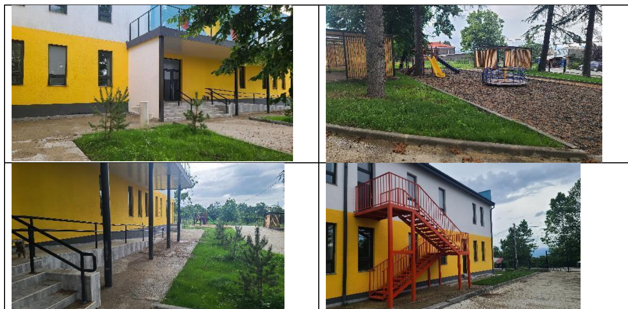
Figure 27 Photo materials reflecting the ongoing civil works
