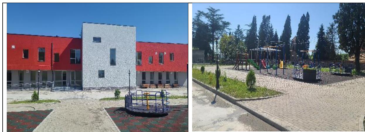
Figure 28 Photo materials reflecting the ongoing civil works
