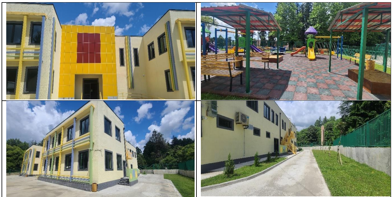
Figure 34 Photo materials reflecting the ongoing civil works
