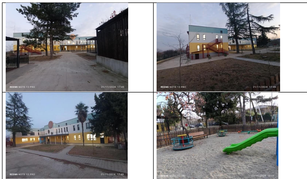
Figure 21 Photo materials reflecting the ongoing civil works
