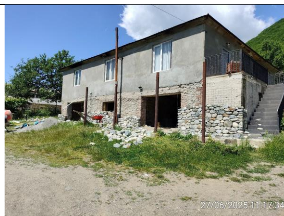
Sector #9 – Building #028 Finishing of the wall in the front façade with stone Dated 23.06.2025
