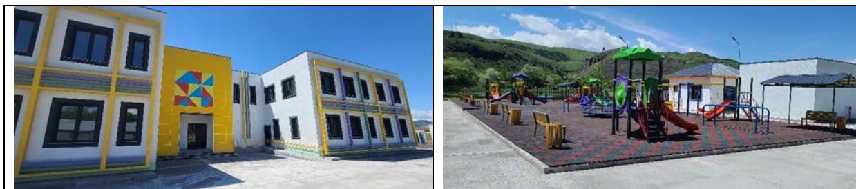
Figure 36 Photo materials reflecting the ongoing civil works
