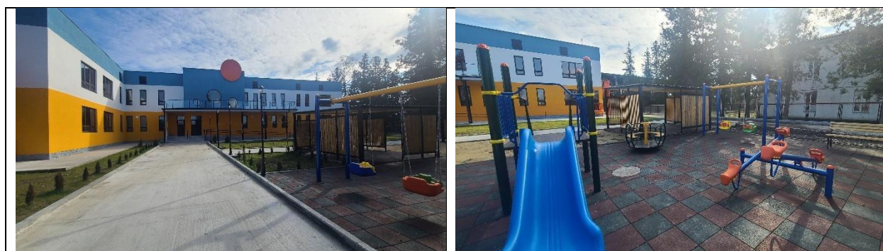
Figure 38 Photo materials reflecting the ongoing civil works
