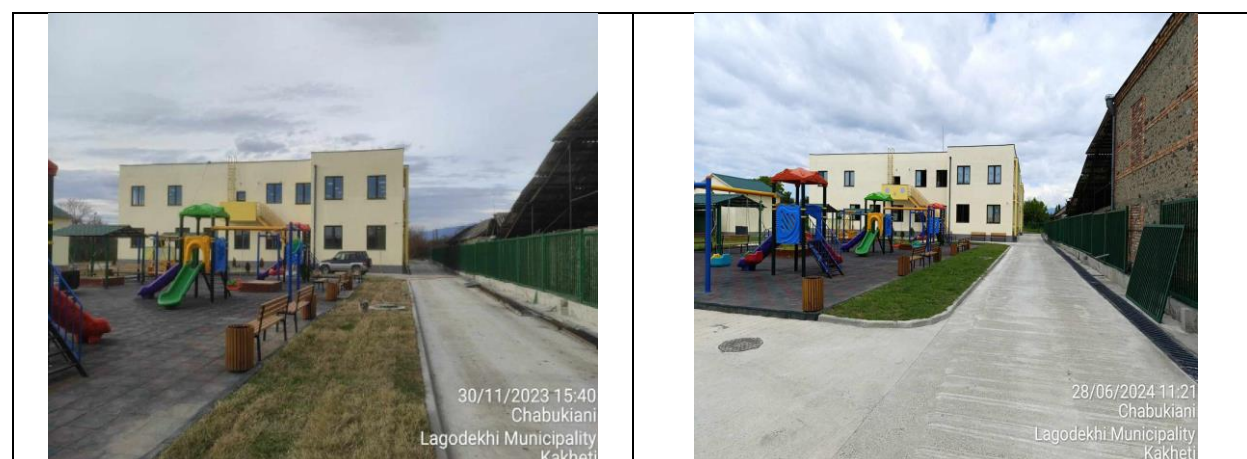
Figure 29 Photo materials reflecting the ongoing civil works
