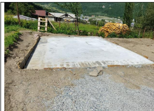
Sector #9 – Building #027 Arrangement of foundation Dated 23.06.2025
