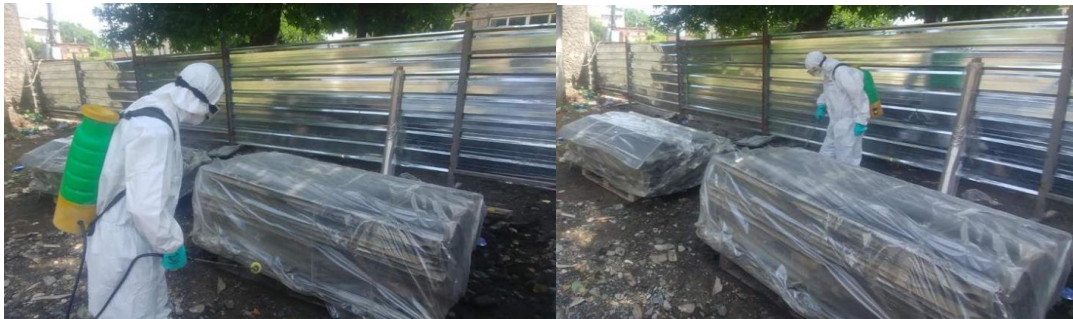
Figure 42. Removal of ACM
