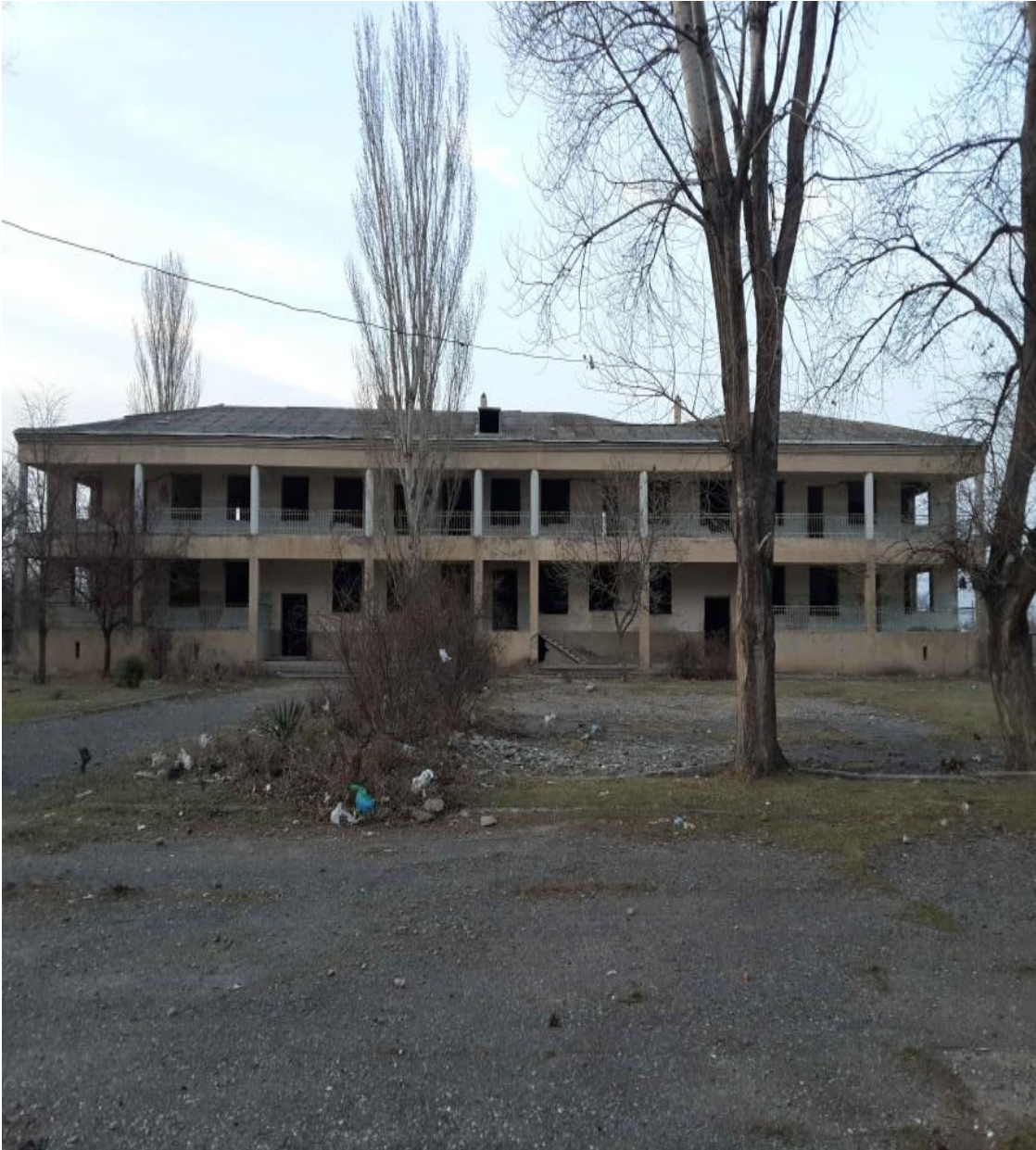
Pictures of the existing building
