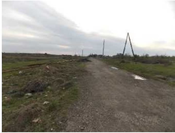
Picture 4.1.3 Pressurized Sewer Corridor
