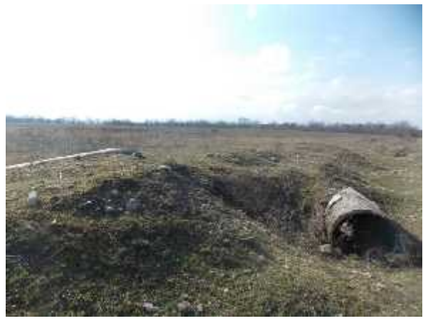
Corridor of the collector
