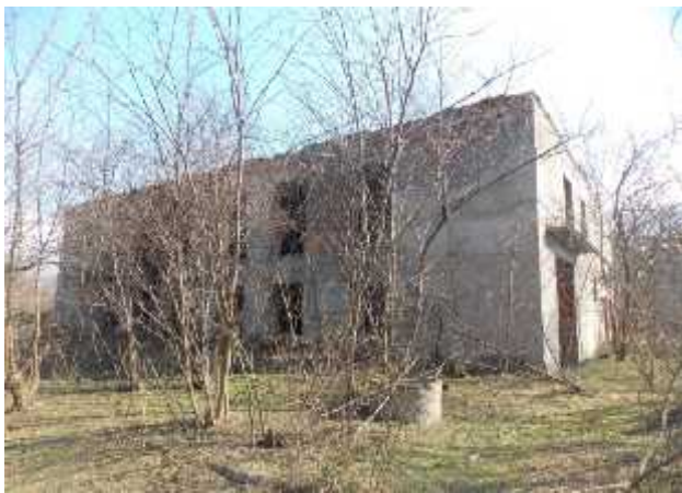
Area for the arrangement of WWTP
