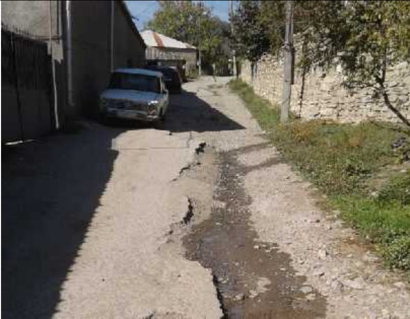
Pictures of the road to be rehabilitated
