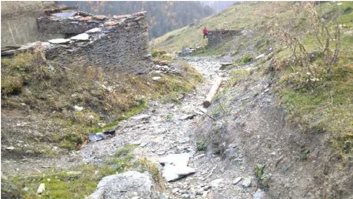
Discharging water from the village to ravine
