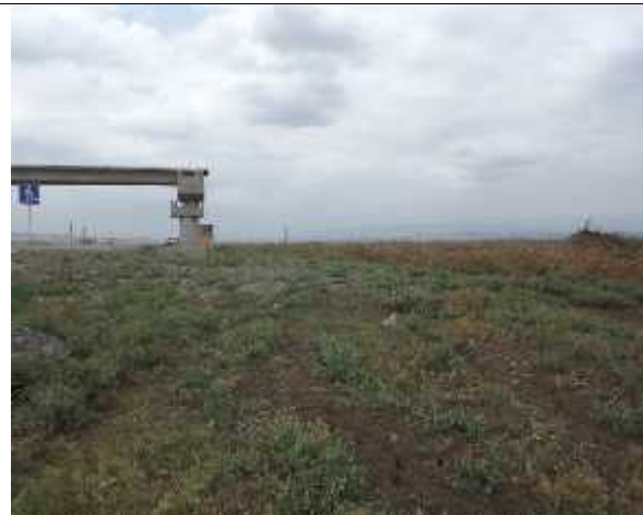
PK 138 Milled asphalt has been removed and used for paving of access roads
