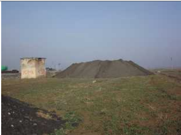
PK 138 Milled asphalt is stored on topsoil
