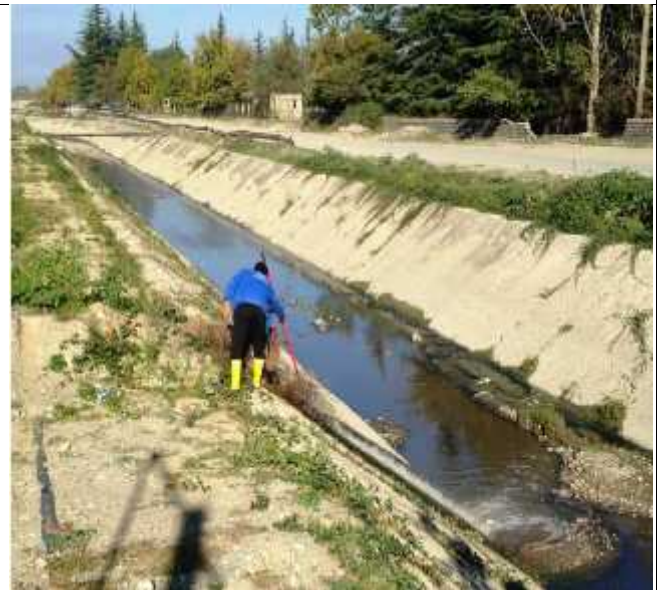
Telavi main sewer draining to irrigation channel
